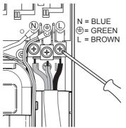
14. Feed cable into case and strip insulation. Firmly connect the conductors. DO NOT exert strain on terminal block.
